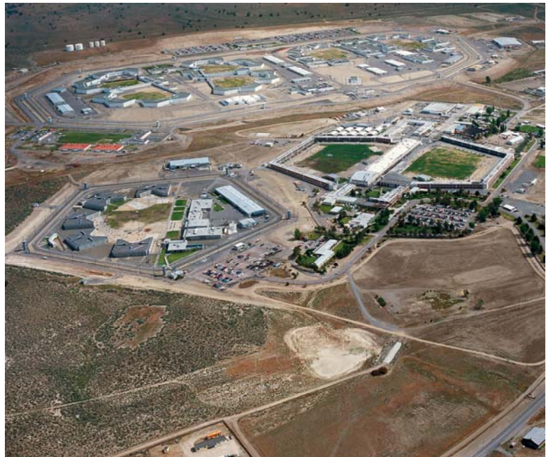
Figure 1 – Aerial view of California Correctional Center
